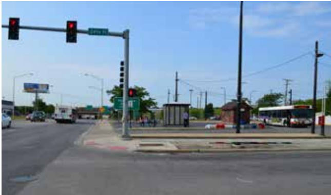
Above: Existing conditions at Cicero Avenue & 24th Place
