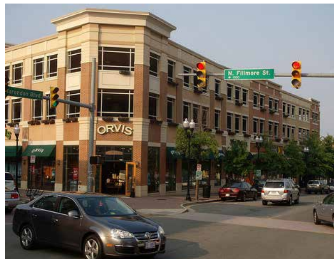
Parking structure with ground floor commercial use
