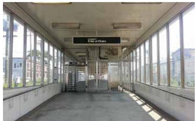
Sign directing transit customers to Cicero Avenue entrance. Source: T.Y. Lin International
