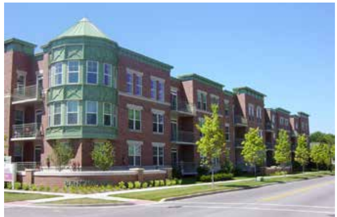
Low-rise multi-family residential building
