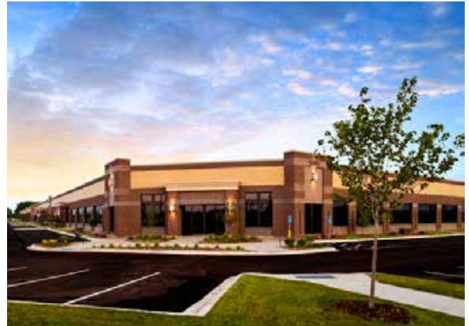
Front office entrance of a manufacturing building
