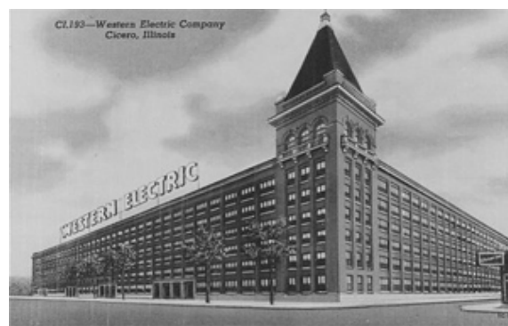
Western Electric Manufacturing Plant
